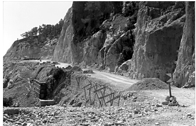
Fig. 6. Landslide problems on a major road constructed through karst towards a proposed hydro-electric development site in southern Turkey. The landslide has occurred at a fault between two limestone units.
